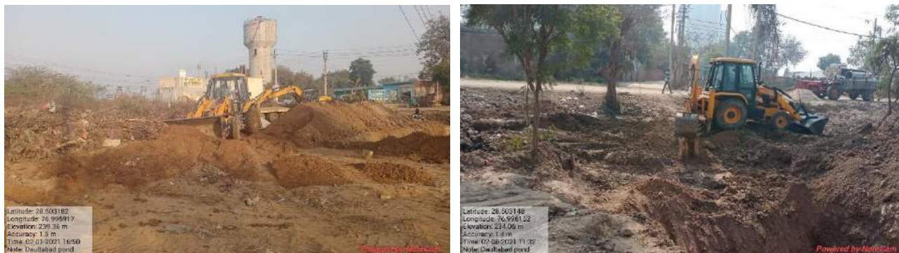
Figure 17: Levelling of Pond
