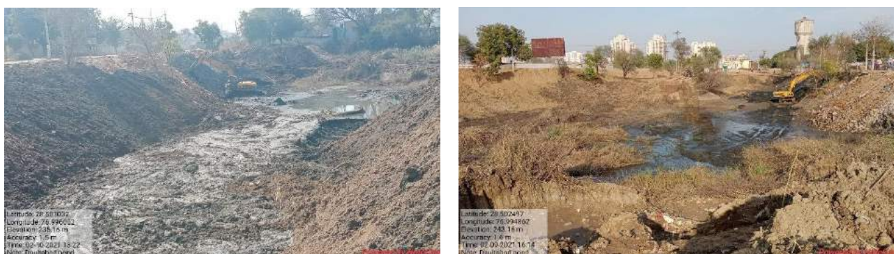
Figure 16: Desilting of the pond
