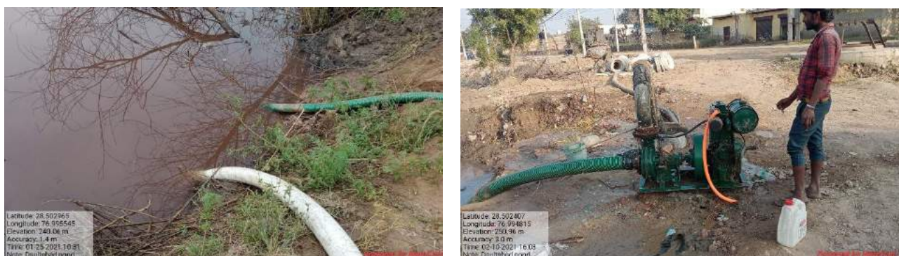
Figure 15: Dewatering of The Pond
