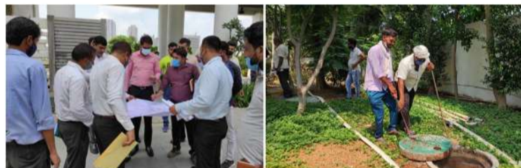
RWH Availability and Functionality Checking by Enforcement Drive Team
