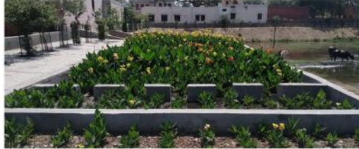
WWTP at Dhaula Pond
