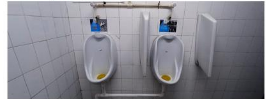
Installation of waterless urinal technology
