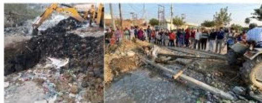
Cleaning work at Gaunchi 146 site
